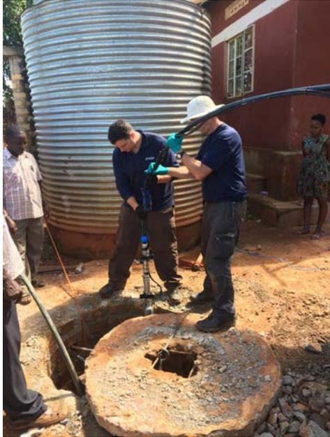
**Wednesday** – time to finish the work started on Tuesday, switch on and test. However, there was a problem... it didn't work! With a little fault finding, quiet contemplation, an open end and change of wiring polarity the pump started with Paul and Keith looking down the open end. I'm not sure if it was the heat or relief but I'm pretty sure they had never been more relieved to get a soaking before.
