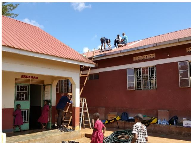
At 48VDC the pump will produce 7b closed head and 1900L/hr. During the day-time we measured the solar panels will produce 69VDC with the controller regulating the supply to the pump. Float switches were fitted to the pump as low-level protection and the storage tank as a pump control.
